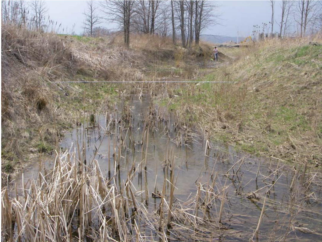
Photo 5. Apr 23, 2007 - View looking upstream immediately downstream of property line. Note the wide, trapezoidal shape of the channel. Also note the extensive vegetative growth on the slopes and channel bed.
