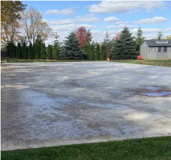
Photo 11. In-season view of concrete pad.
