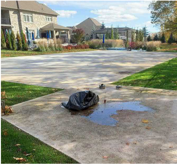
Photo 9. In-season view of concrete pad.
