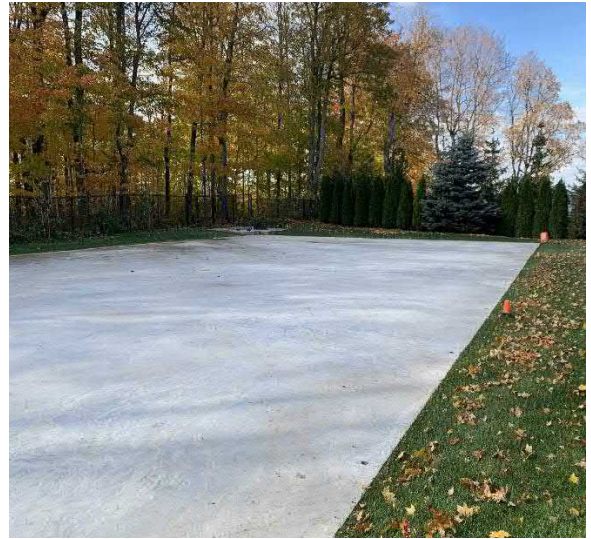
Photo 10. In-season view of concrete pad.
