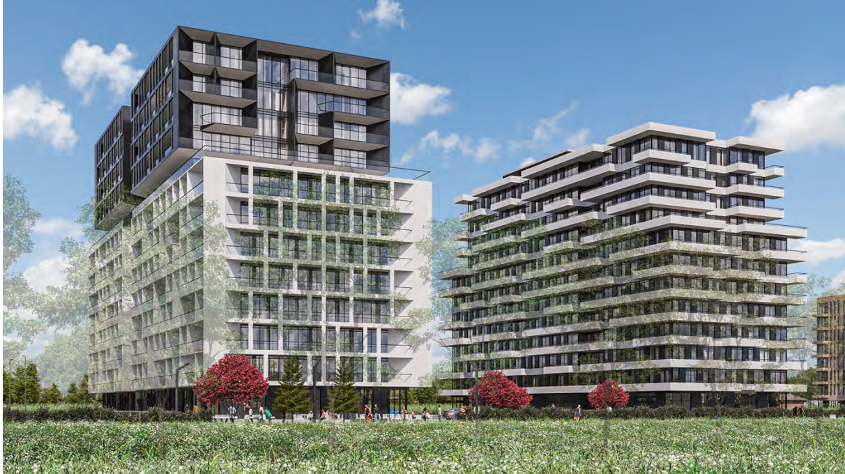
Figure 3 View from the North West, North Block (CORE Architects)
