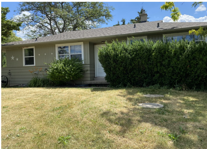
PHOTO 17: View of septic tanks located adjacent to the north portion of Site Building D.
