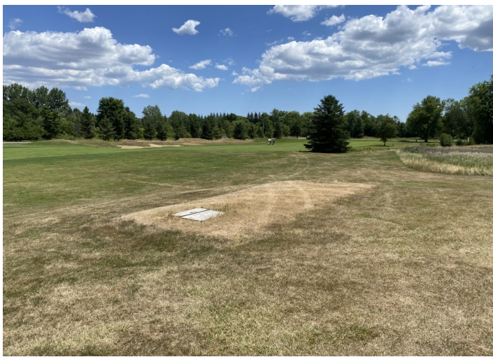
PHOTO 7: View of a septic tank located approximately 20 m east of Site Building B.
