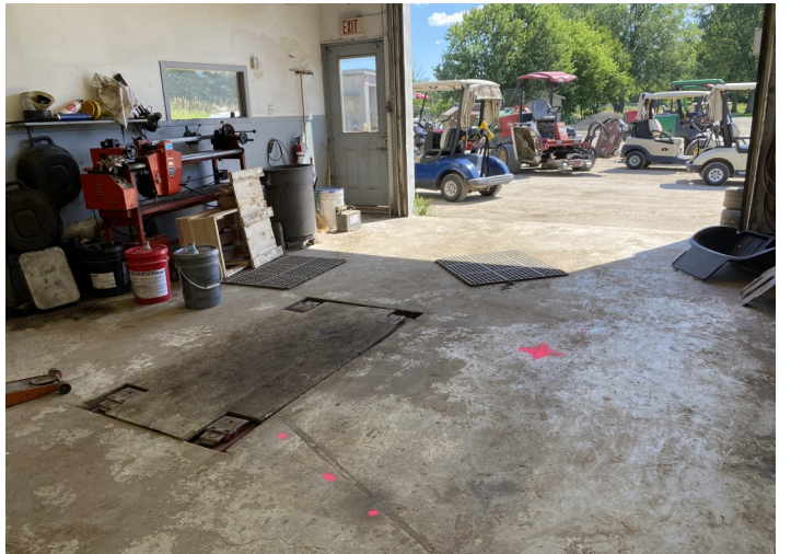
PHOTO 10: View a hydraulic lift located in Site Building C.
