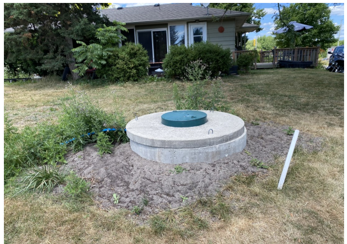
PHOTO 18: View of water well located 10 m south of Site Building D.
