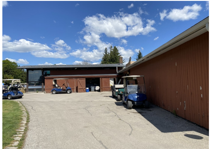
PHOTO 2: View of the western portion of Site Building B, facing north.
