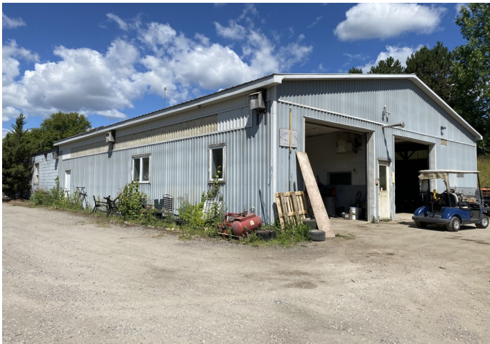
PHOTO 3: View of eastern and southern portions of Site Building C, facing northwest.
