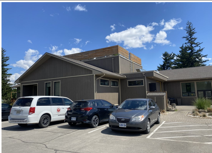
PHOTO 1: View of the western portion of Site Building A, facing east.
