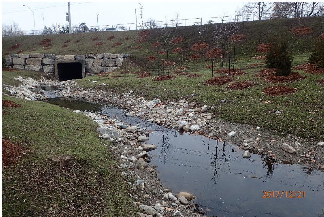
Looking at channel downstream of outfall location. Note the newly constructed channel with riffle-pool sequences.
