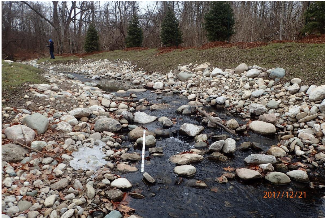
Looking upstream of unnamed tributary. Note the stable channel banks. No erosion was present along the tributary downstream of the proposed outlet.
