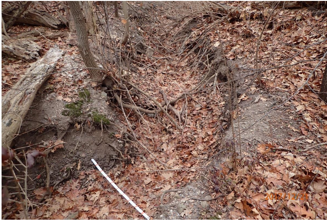
Looking at approximate outfall location for the stormwater management outlet.
