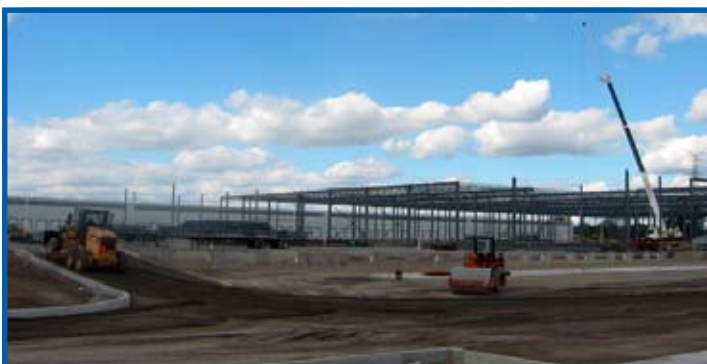
SYSCO Canada facility under construction
