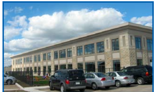
Bronte Street Professional Centre Building one of three planned
