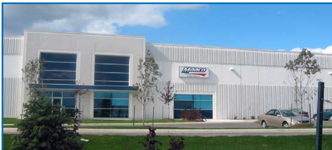
Maaco Systems Canada head office
