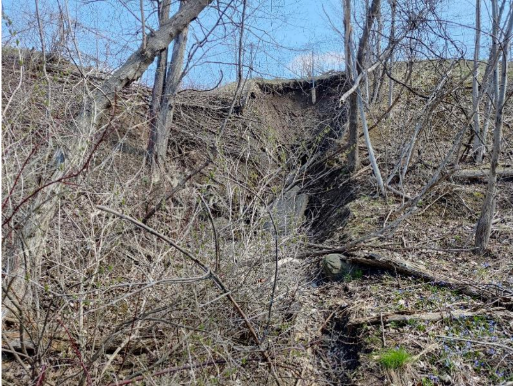
Photo 5: Slope conditions and erosion/failure in Cross-Section B-B area (looking north from toe of slope)
