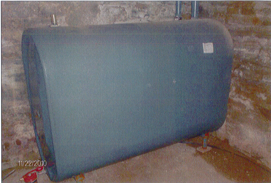
View of AST located in the basement of the home on the subject site
