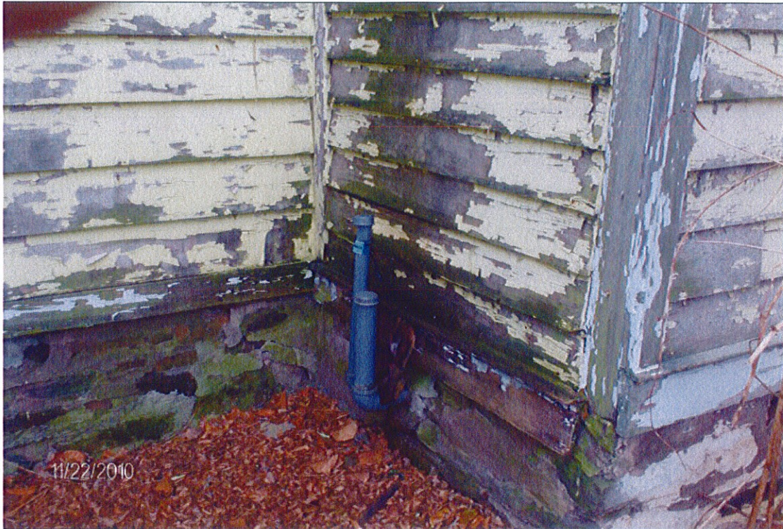
View of vent and fill pipes located on the eastern wall of the home
