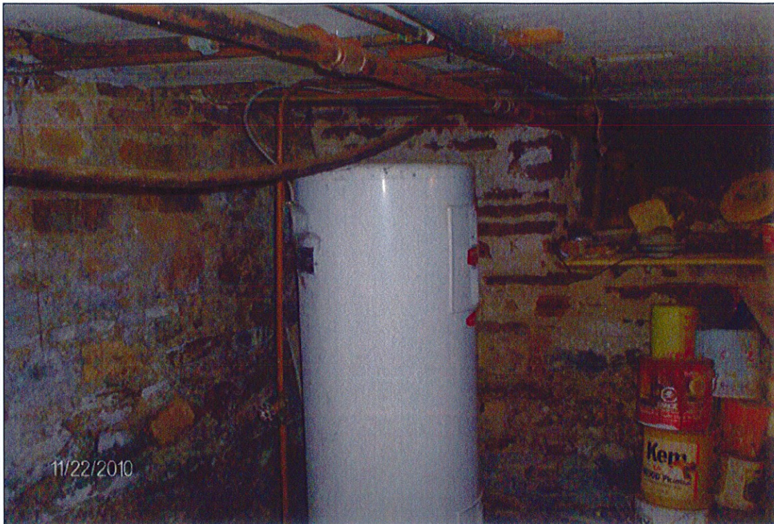
View of electric hot water heater located in the basement of the home
