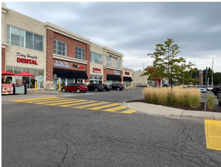
Photo 2 – Generally view of the 6941 Derry Road, facing northeast
