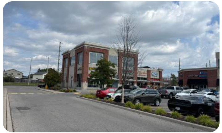
Existing Building “D”
