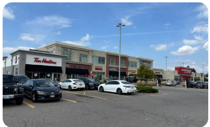
Existing Building "C"
