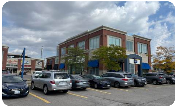
Existing Building “E”
