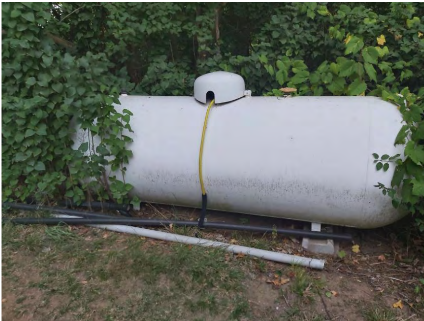
Looking at the propane AST located on the subject site
