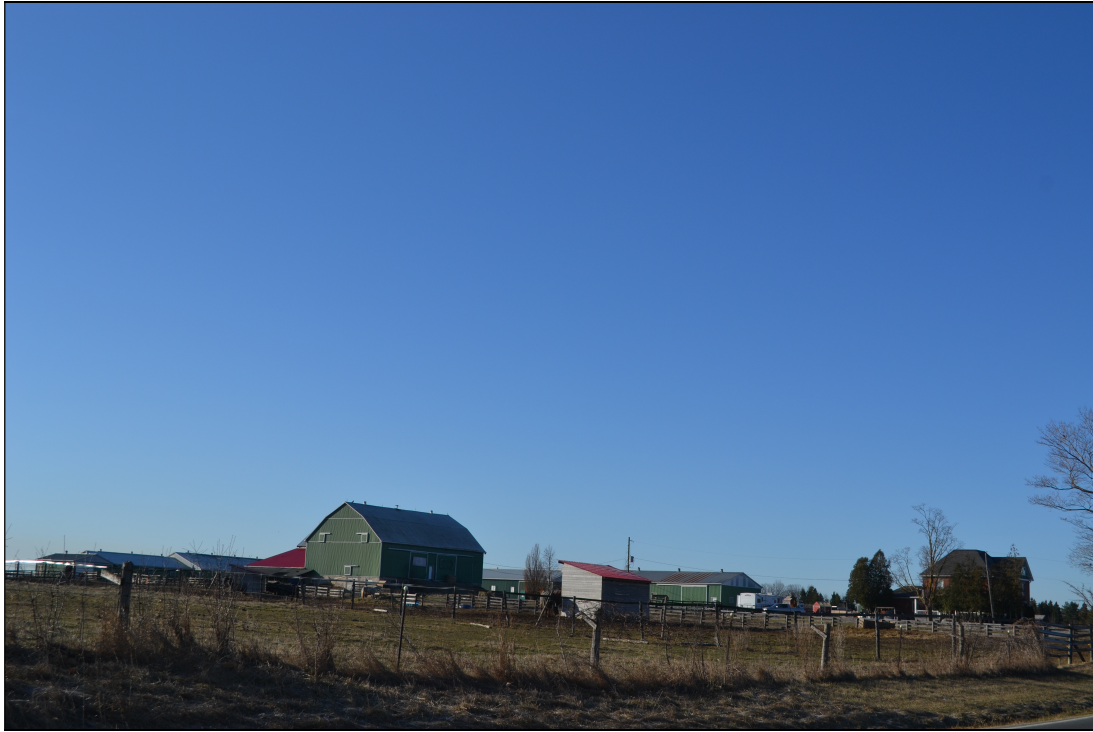
Attachment E, Photo 11: Barn B11
