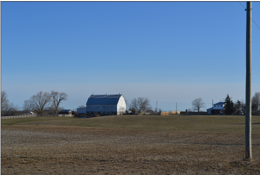
Attachment E, Photo 10, Barn B10
