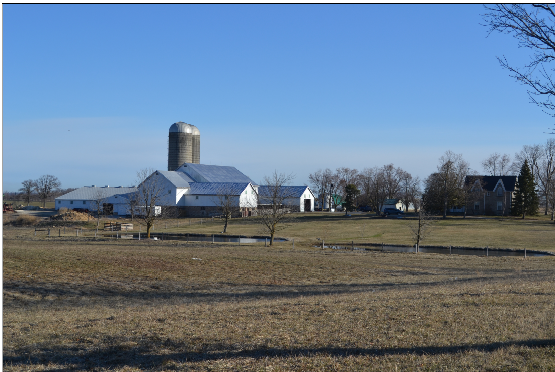
Attachment E, Photo 12: Barn B12
