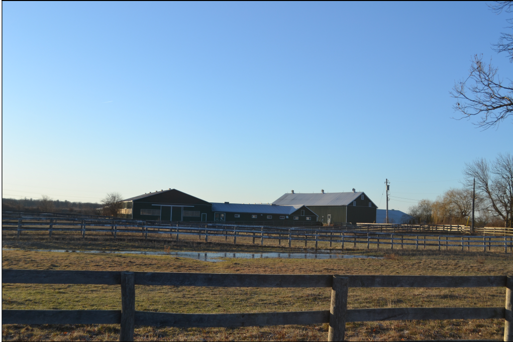
Attachment E, Photo 1: Barn B1
