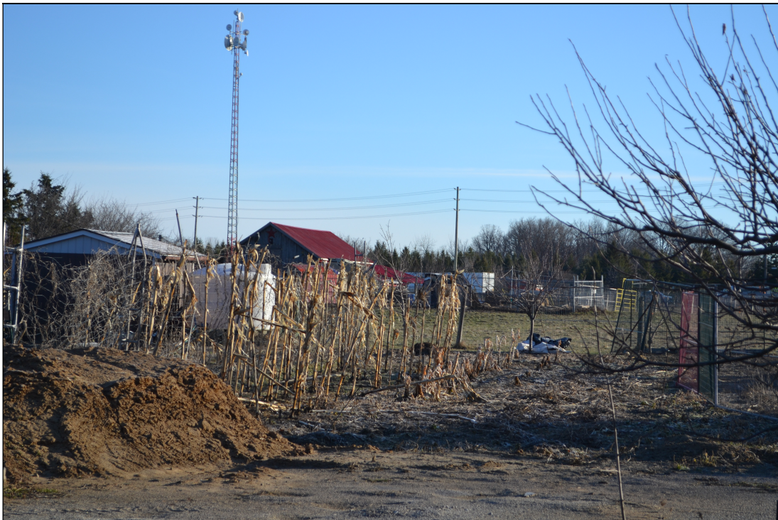
Attachment E, Photo 6: Barn B6
