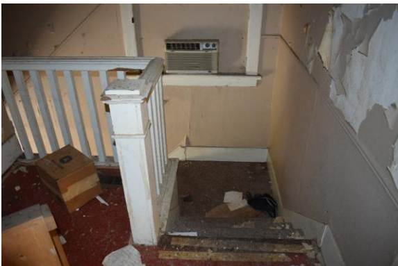
Photo 117: Staircase from second storey, looking south
