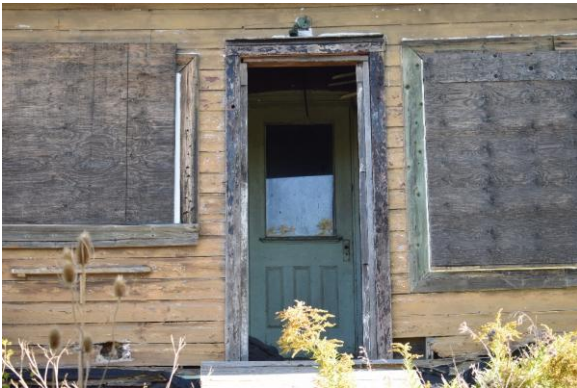
Photo 107: Rear enclosed porch and entrance, looking east
