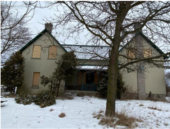
Photo 24: Rear elevation, looking east
