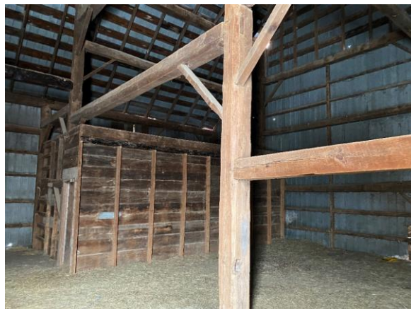
Photo 85: Upper storey, looking northwest
