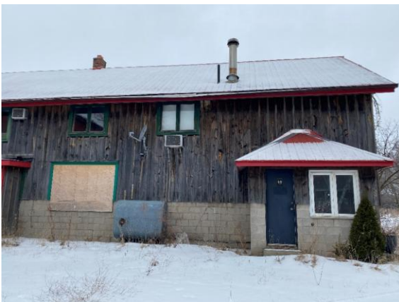
Photo 76: Barn addition, looking north
