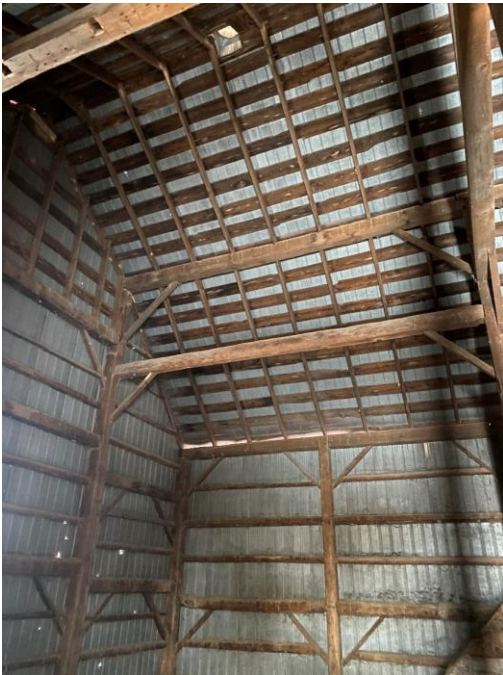
Photo 86: Wood timber frame and rafters, looking southwest
