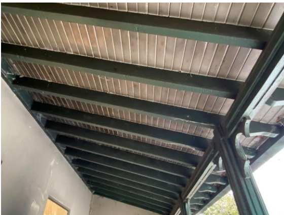
Photo 26: Rear porch roof, looking south
