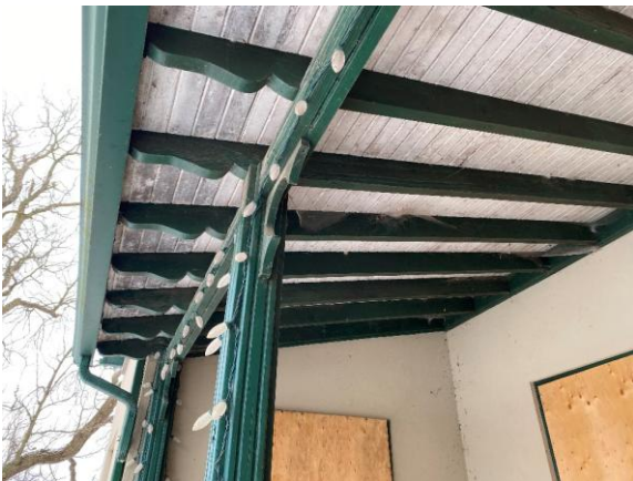
Photo 22: Front porch roof, looking south
