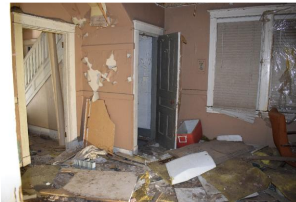
Photo 115: Kitchen, looking southeast
