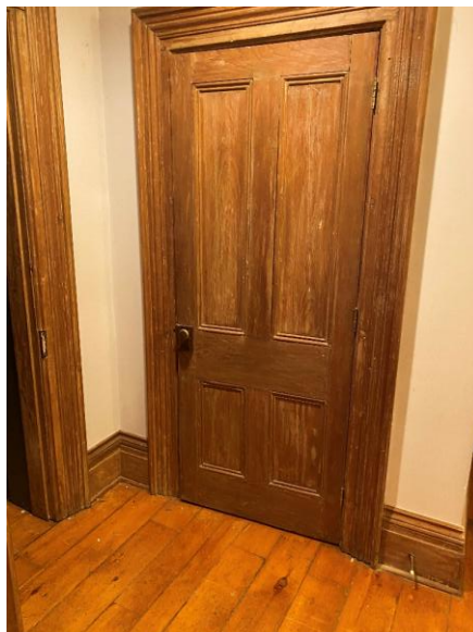
Photo 57: Upstairs hall closet door, looking southwest
