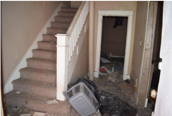
Photo 109: Central hallway, looking west
