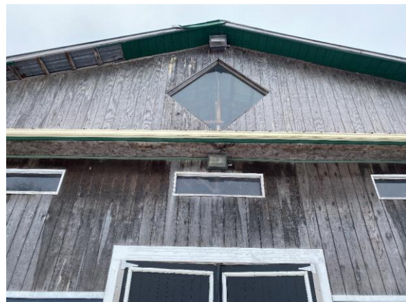
Photo 93: Riding Arena north gable windows
