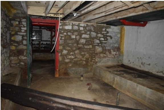
Photo 62: Basement central portion, looking northeast
