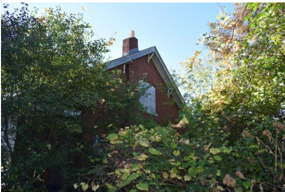
Photo 105: North elevation, looking southwest
