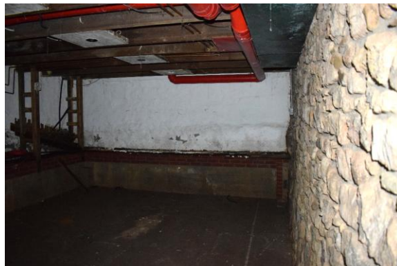
Photo 65: Basement north portion, looking east
