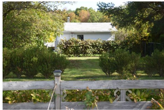
Photo 4: Rear outbuilding, looking east
