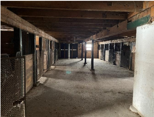
Photo 78: Lower storey, looking south
