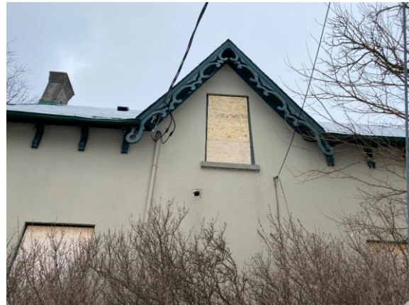
Photo 29: South elevation gable peak
