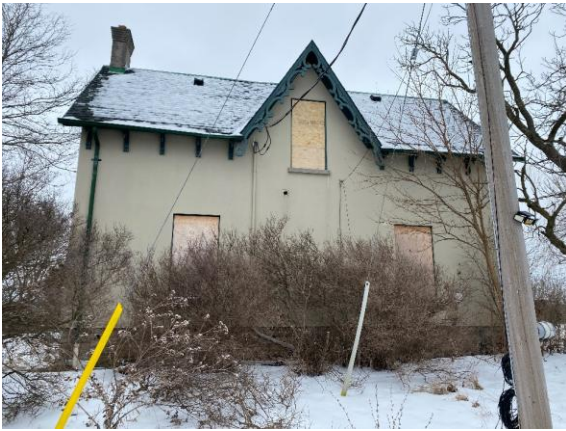
Photo 28: South elevation, looking northeast
