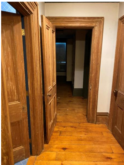
Photo 56: Upstairs hallway, with south bathroom on left, bedroom/dressing room at end of hall, and closet on right, looking south
