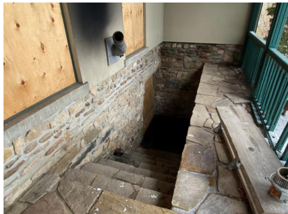
Photo 27: Basement access, looking south
