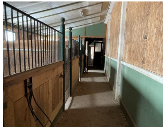
Photo 97: Stables, looking north
