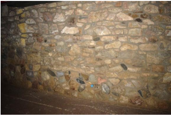
Photo 66: Basement north portion rubble stone wall, looking southeast
