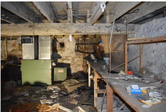
Photo 123: Basement, looking north
