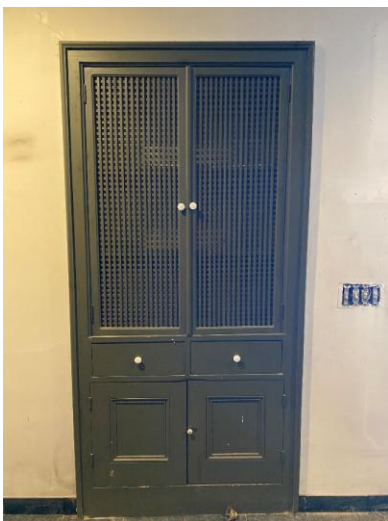
Photo 40: Kitchen built-in, looking south
