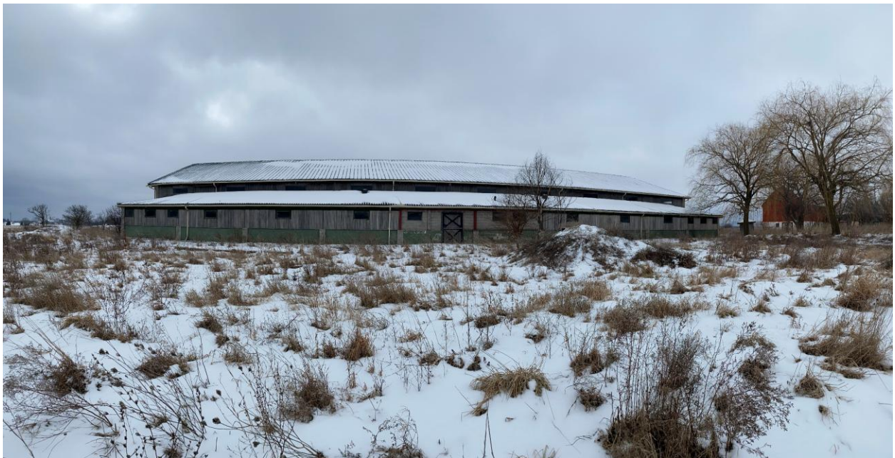
Photo 89: Riding Arena, looking west
