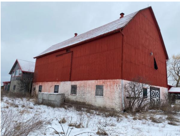
Photo 72: Barn, looking northeast
