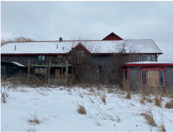
Photo 74: Barn addition, looking south
