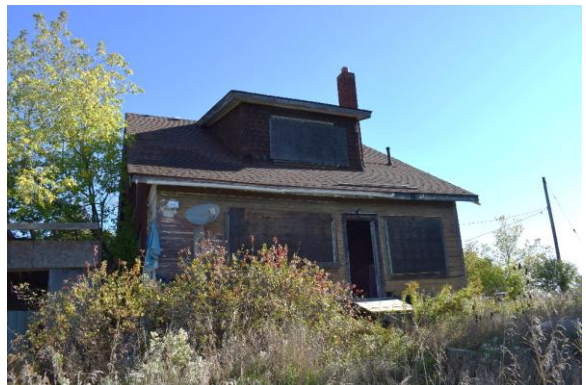
Photo 106: West elevation, looking southeast
