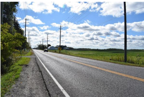
Photo 1: Tremaine Road, looking southwest
