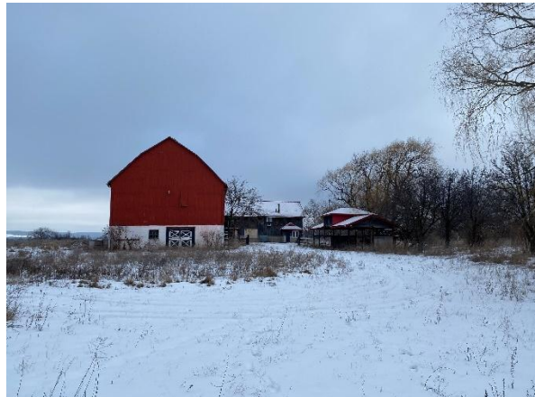
Photo 71: Barn, looking north
