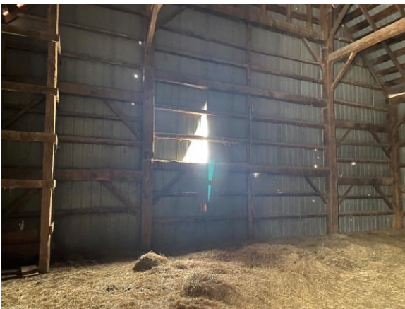
Photo 84: Upper storey, looking southwest
