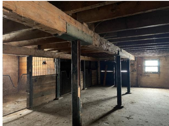
Photo 79: Lower storey, looking southeast
