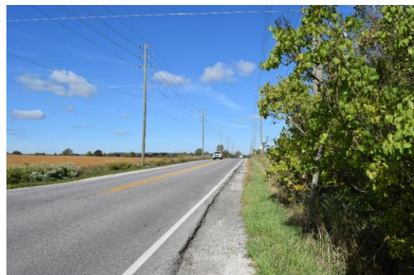
Photo 2: Tremaine Road, looking north
