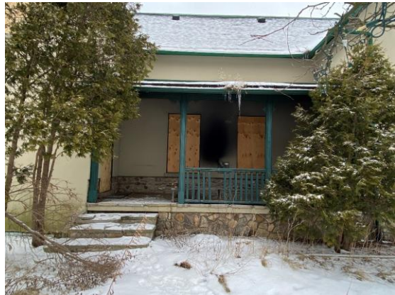
Photo 25: Rear porch, looking east
