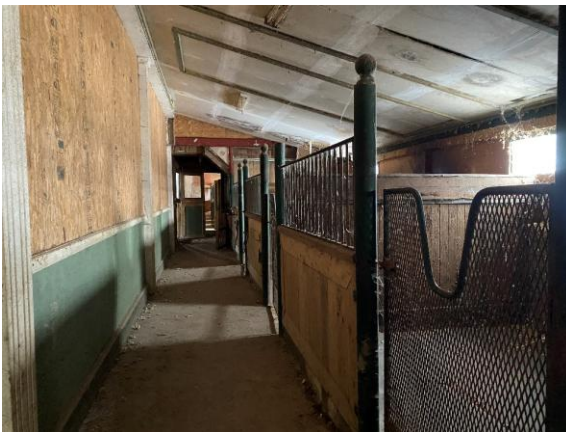
Photo 96: Stables, looking south
