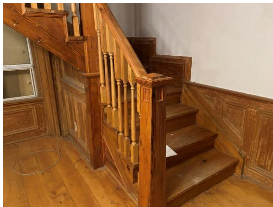
Photo 33: Central front hall staircase with boxed newel
