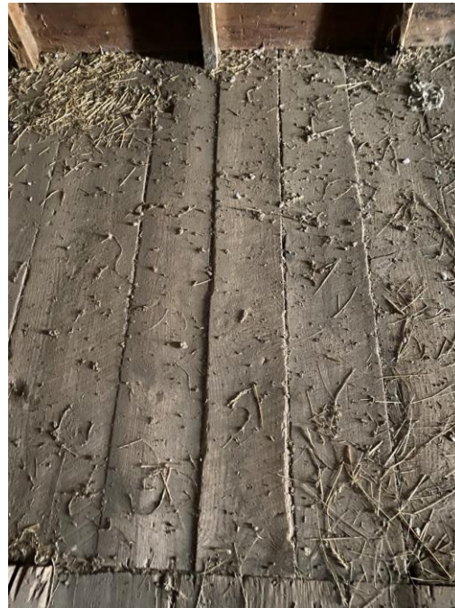
Photo 87: Close-up of wood flooring
