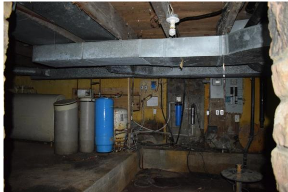
Photo 63: Basement south portion, looking south
