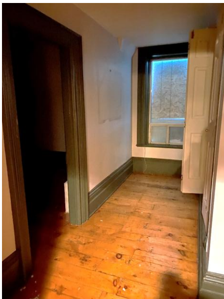
Photo 60: South dressing room, looking south
