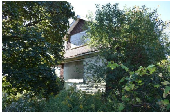
Photo 104: Front façade, looking southwest
