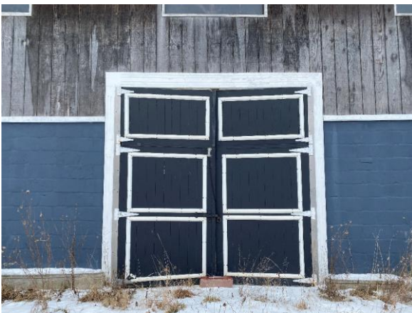
Photo 92: Riding Arena north entrance doors, looking south
