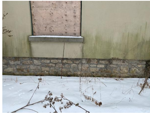
Photo 19: Close-up of foundation
