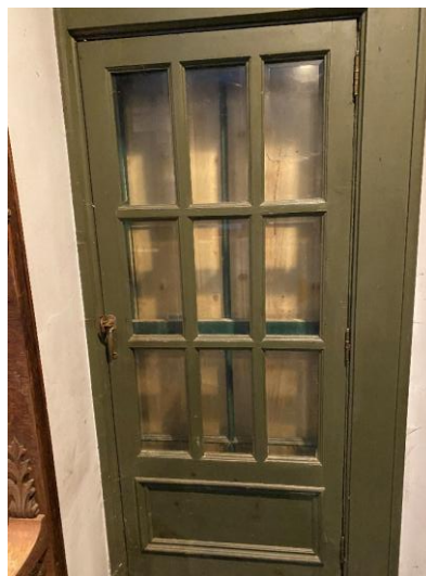
Photo 41: Kitchen door over exterior window, looking west
