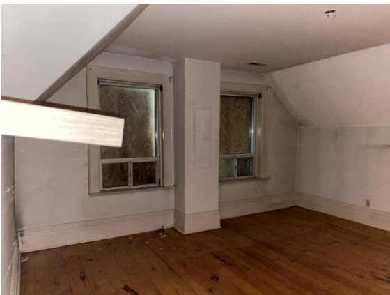
Photo 52: North bedroom, looking northwest
