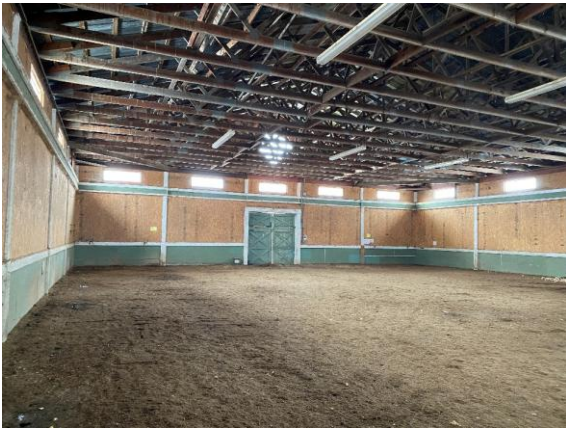
Photo 94: Riding Arena, looking northeast
