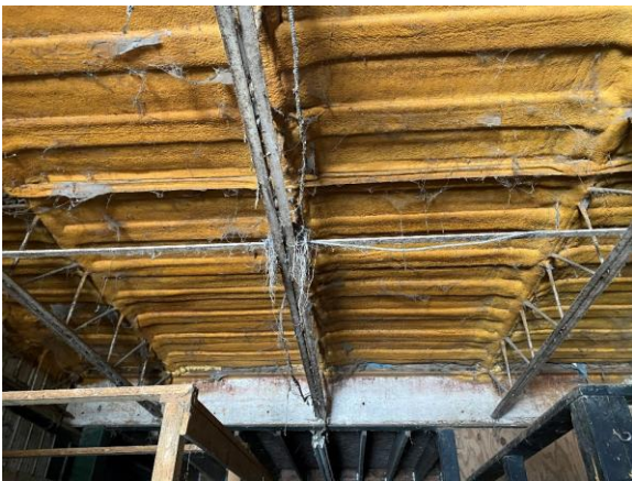
Photo 82: Close-up of lower storey addition ceiling
