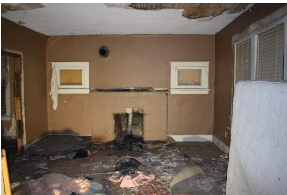
Photo 111: Living room, looking north
