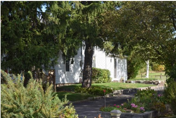
Photo 7: South elevation, looking northeast
