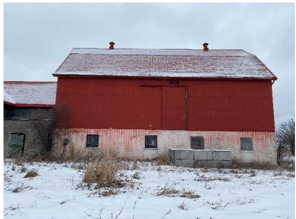
Photo 73: Barn, looking east
