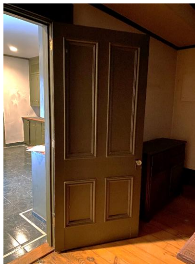
Photo 37: Dining room door off kitchen, looking northwest
