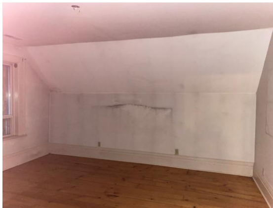
Photo 51: North bedroom, looking north
