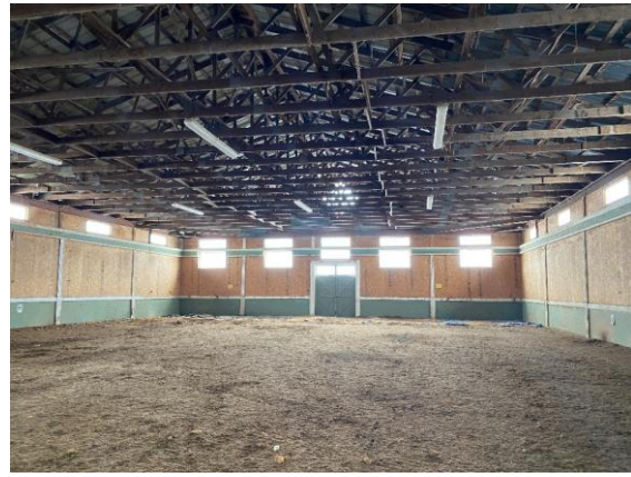
Photo 95: Riding Arena, looking southeast
