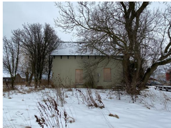
Photo 23: North elevation, looking south
