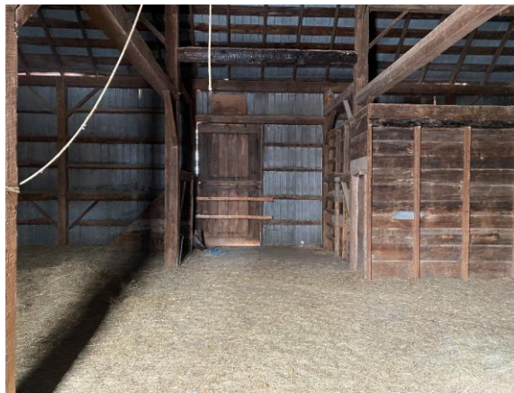
Photo 83: Upper storey, looking west
