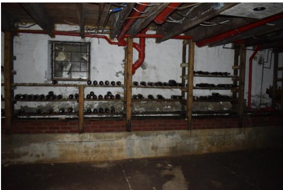
Photo 64: Basement north portion, looking north
