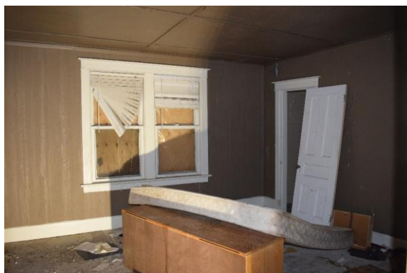
Photo 120: North bedroom, looking northeast
