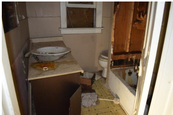
Photo 118: Bathroom, looking southwest
