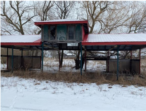
Photo 16: Equestrian outbuilding, looking south
