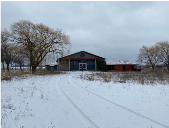
Photo 90: Riding Arena north elevation, looking south
