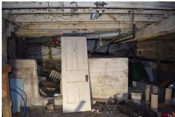
Photo 124: Basement, looking west
