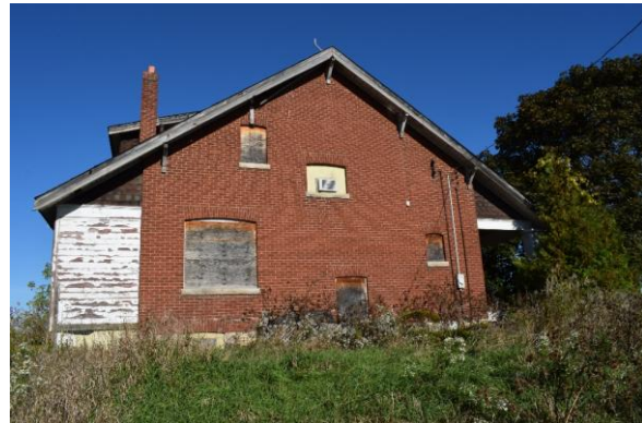
Photo 108: South elevation, looking northeast
