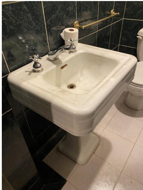
Photo 47: Close-up of powder room sink, looking northwest
