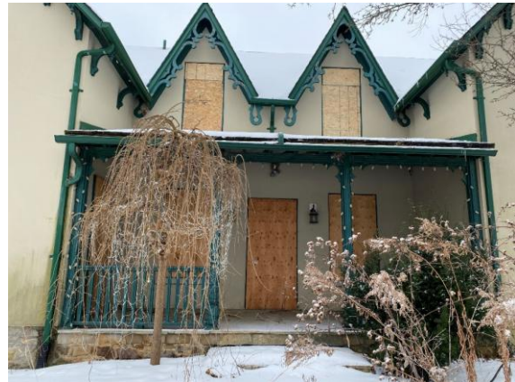
Photo 21: Front façade porch, looking west
