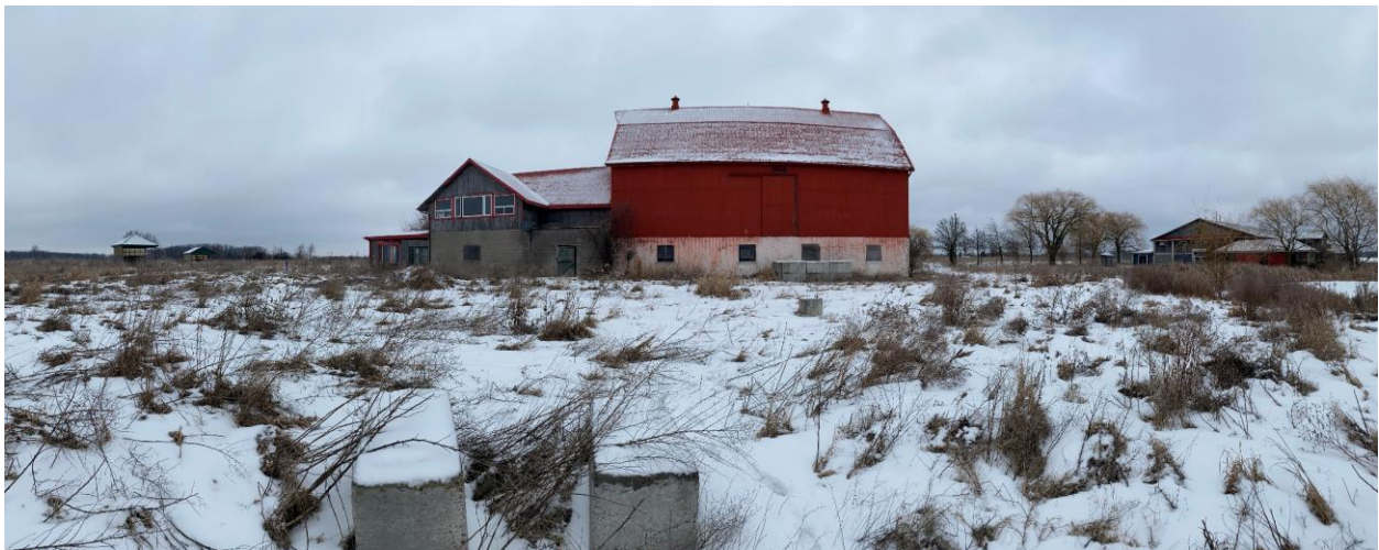
Photo 69: Barn, looking east
