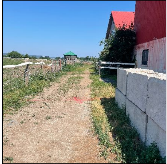
Image 14: Area of disturbance, note high voltage utilities.
