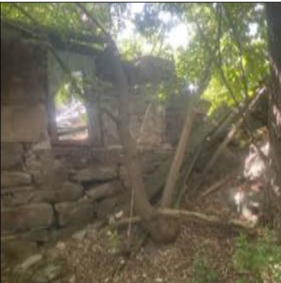
Image 31: Example of ruined barn noted within the Study Area.
