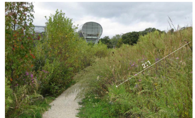
Lake Whitney Water Treatment Facility, Connecticut
