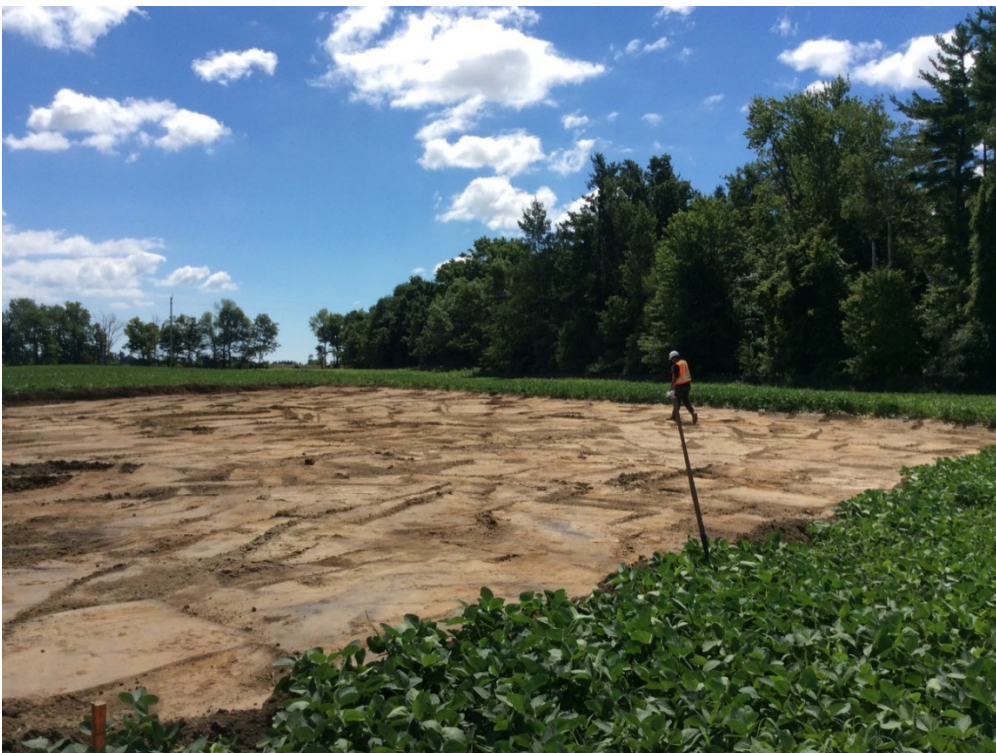
Image 4: Stage 4 mechanical topsoil removal, inspection subsurface interface for cultural features, facing southwest
