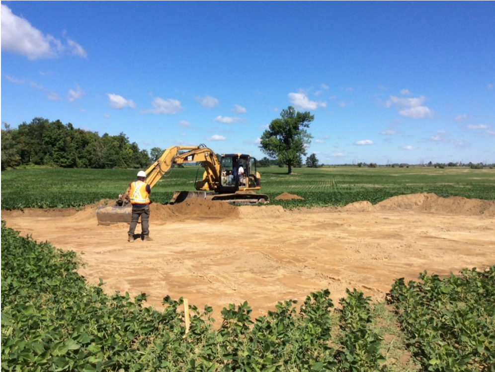
Image 3: Stage 4 mechanical topsoil removal in progress, facing southwest
