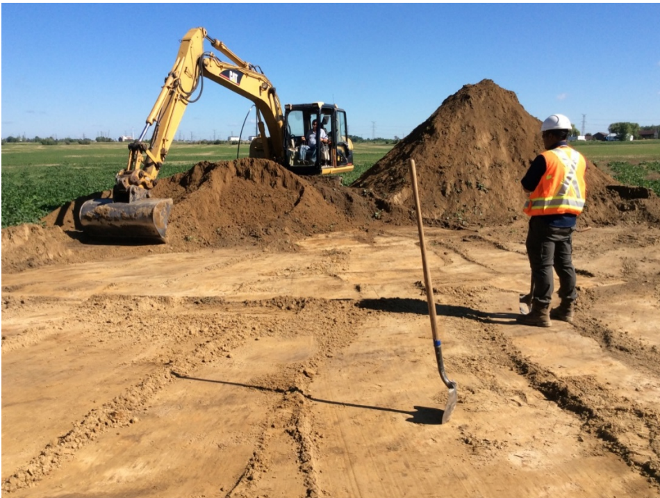
Image 2: Stage 4 mechanical topsoil removal in progress, facing north
