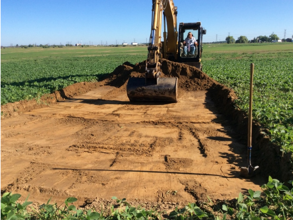
Image 1: Stage 4 mechanical topsoil removal in progress, facing north
