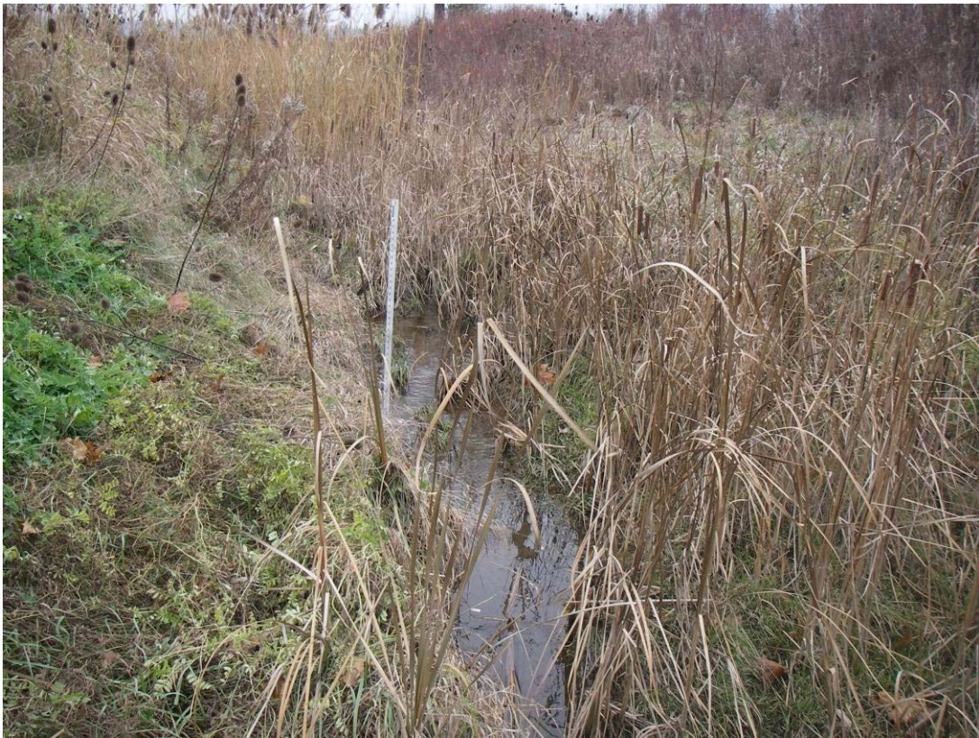
Photo 1. Nov 14, 2006 - View of channel conditions of Tributary N1-A adjacent to Highway 401. Note the dense vegetation and trapezoidal shape of the channel
