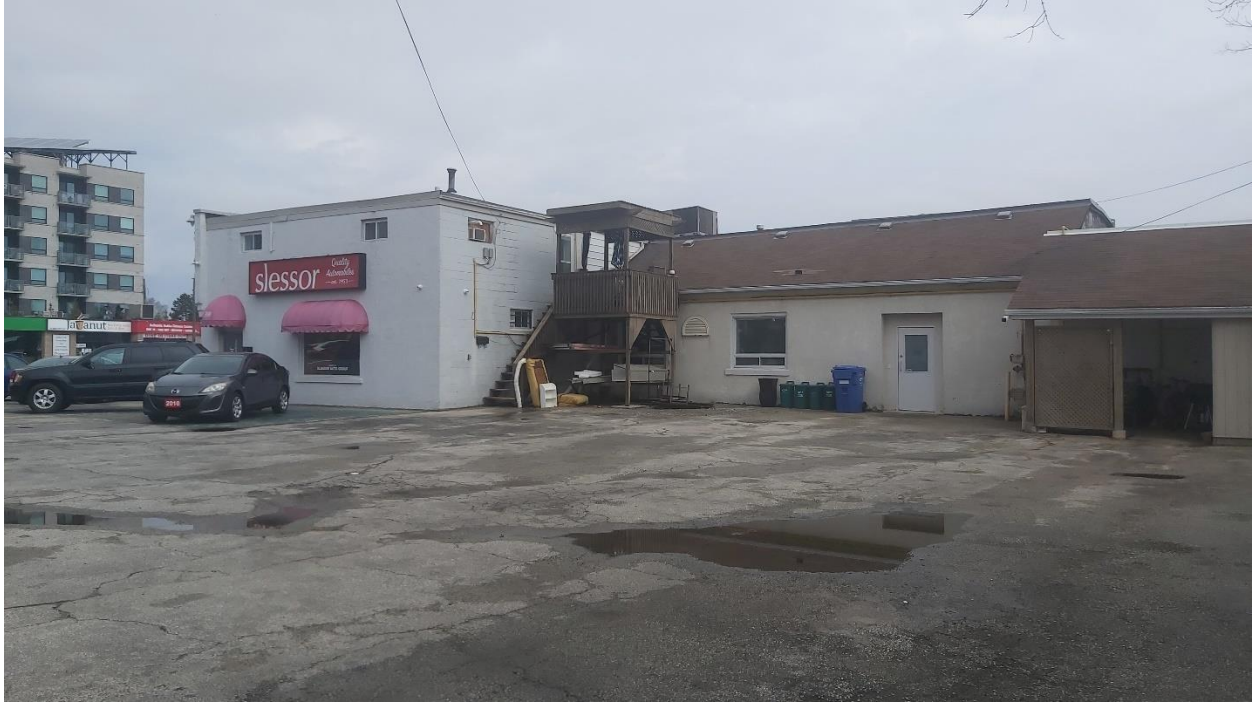
Photo of the west side of the commercial/residential building at 388 Main Street East. Taken from the western portion of the Site, facing northeast.
