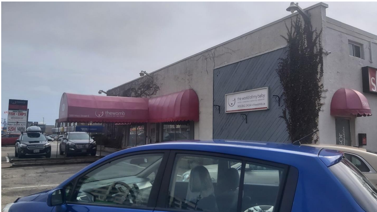
Photo of the north side of the commercial/residential building at 388 Main Street East. Taken from the northern portion of the Site, facing southeast.
