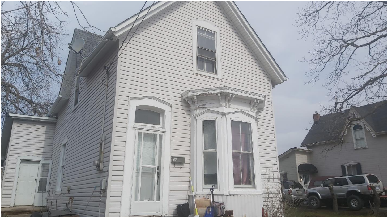
Photo of the south side of the dwelling at 395 Pearl Street. Taken from the southern portion of the Site, facing north.
