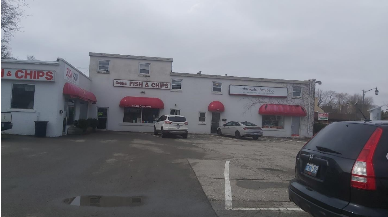
Photo of the east side of the commercial/residential building at 388 Main Street East. Taken from the eastern portion of the Site, facing west.
