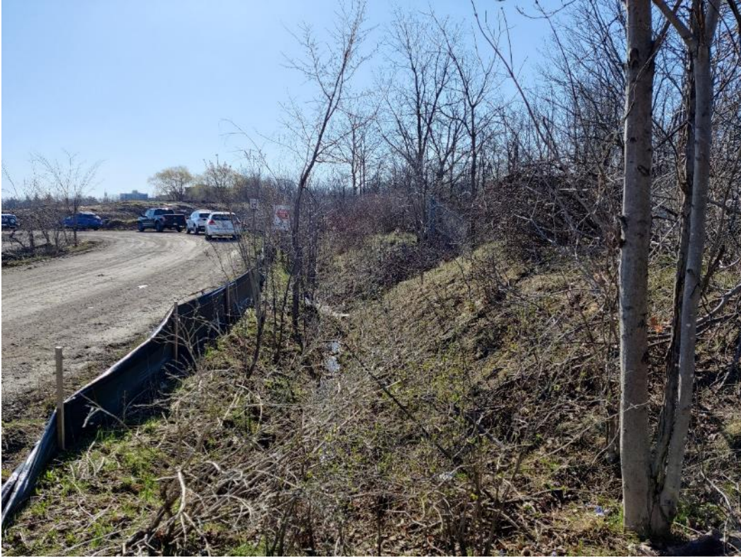
Photo 1: Top of Slope Area in Cross-Section B-B and C-C (looking east)
