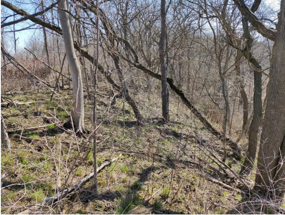
Photo 17: Top of slope conditions in middle area between Cross-Sections G-G and H-H (looking east from top of slope)
