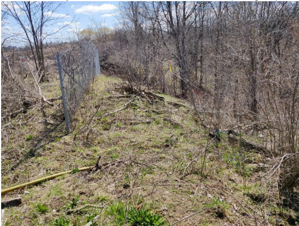
Photo 2: Slope Condition in Cross-Section B-B and C-C Area (looking east)
