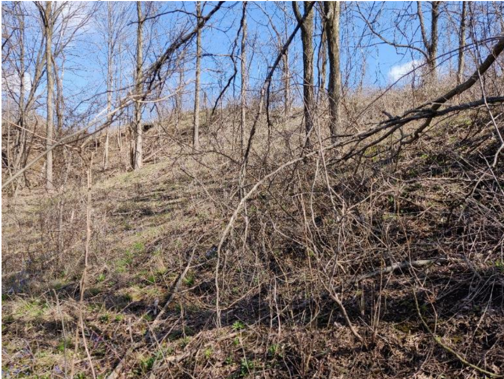
Photo 12: Slope conditions in Cross-Sections D-D to E-E area (looking northwest from toe of slope at east of Cross-Section E-E)
