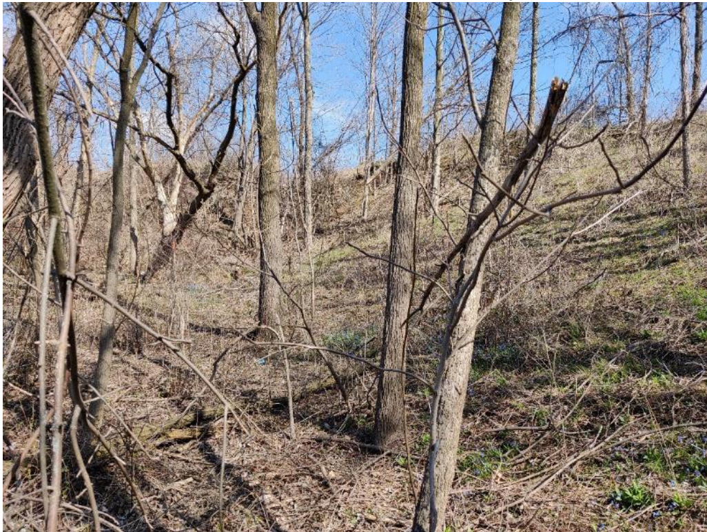
Photo 4: Slope Conditions in Area of Cross-Sections A-A to C-C (looking northwest from toe area of slope)
