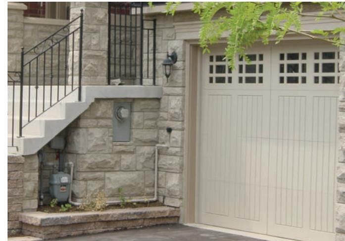
For Townhouses and other higher density forms, utility meters should be architecturally integrated or screened
