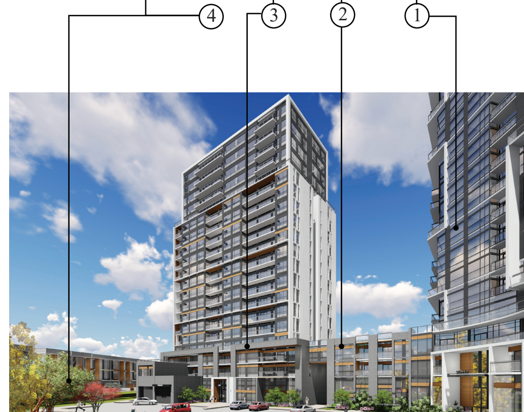
CONDOMINIUM BUILDINGS : VIEW OF BUILDING "A" FROM BUILDING B DROP-OFF
