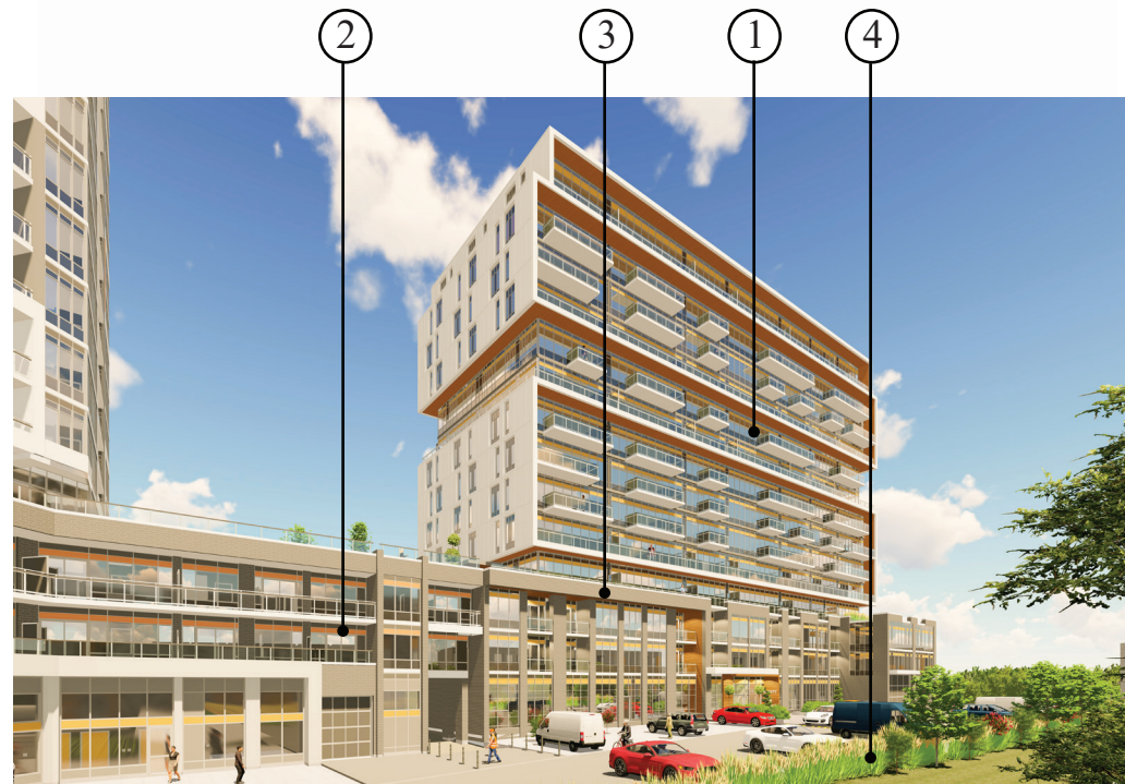
CONDOMINIUM BUILDINGS : VIEW OF BUILDING "C" FROM BUILDING "B" ENTRANCE
