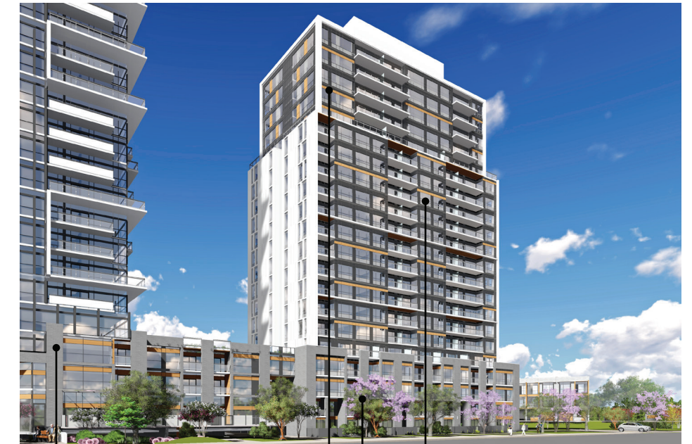
CONDOMINIUM BUILDINGS : BUILDING "A" FROM REGIONAL ROAD 25
