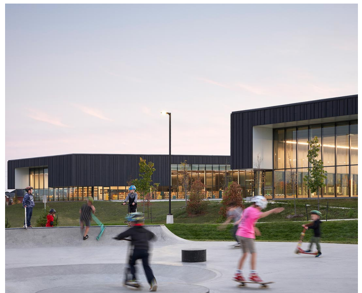
Sherwood Community Centre and Library, Milton
