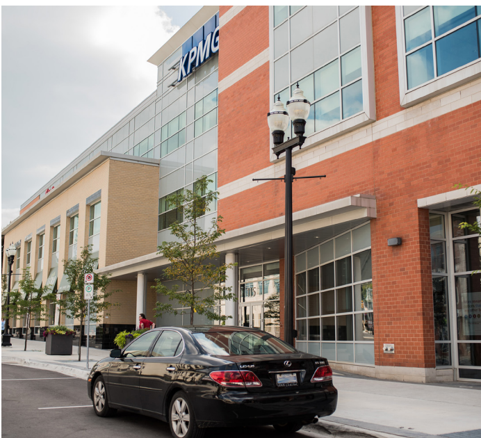
On-Street Parking should be provided along the Enhanced Streetscape
