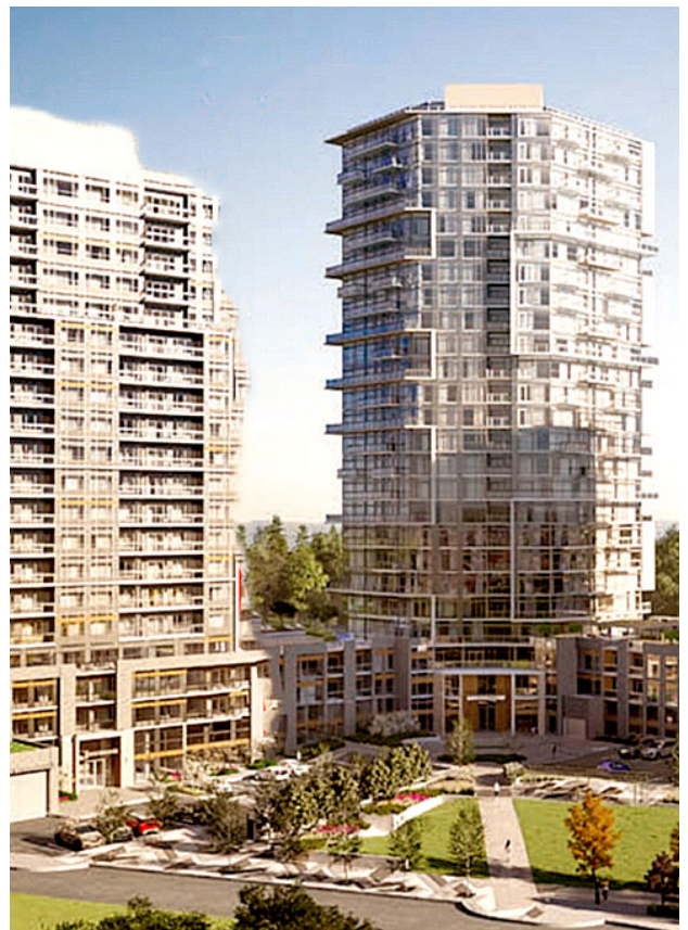
Break up the building mass with changes in material, balconies, setbacks and building articulation
