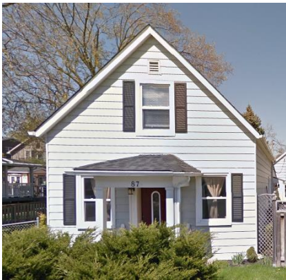
Example of Regency Cottage Style
