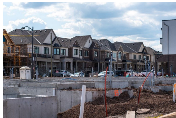
Figure 41. Construction site in Milton (Town of Milton files).
